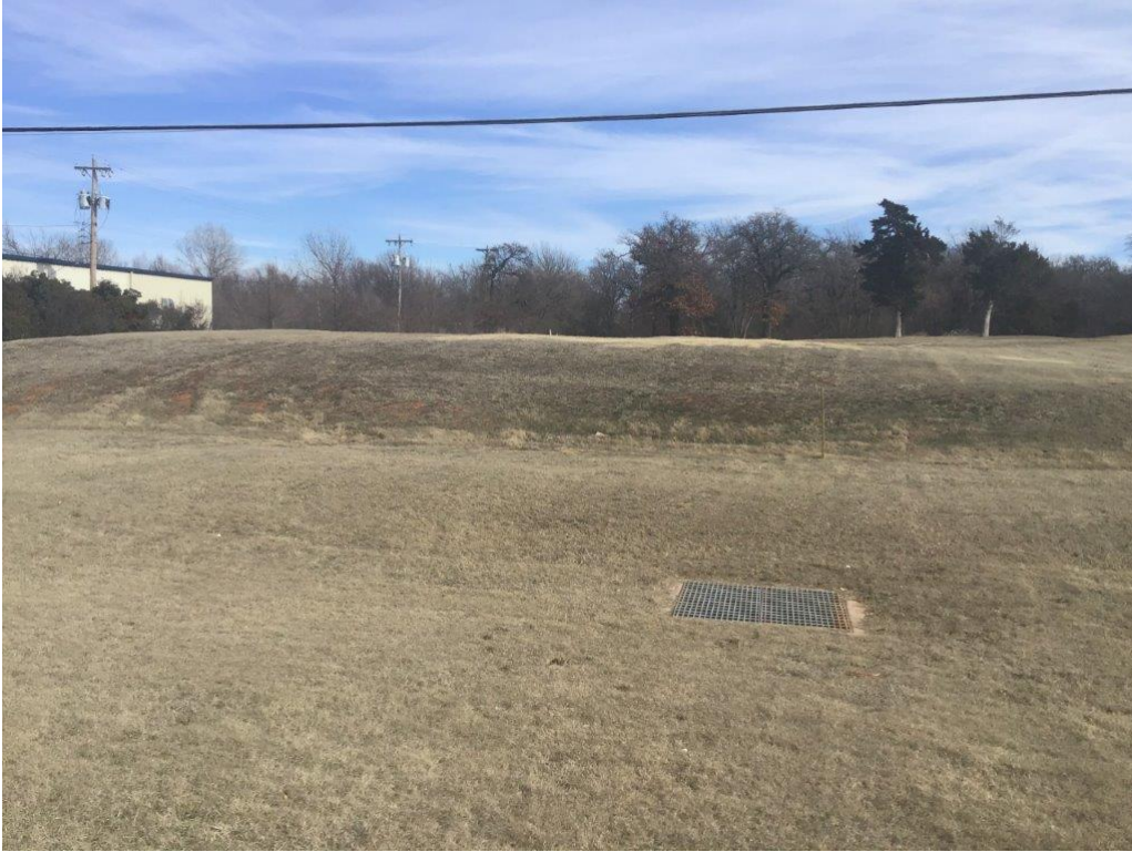
View looking from frontage east towards Lot 1. Propose outflowing detention pond to this existing inlet.
