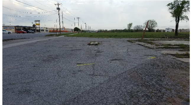
Photo #2: Dispenser Island : Pre-Excavation
