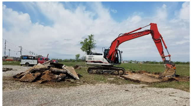
Photo #6: Tank #1 and #2 Pit Excavation
