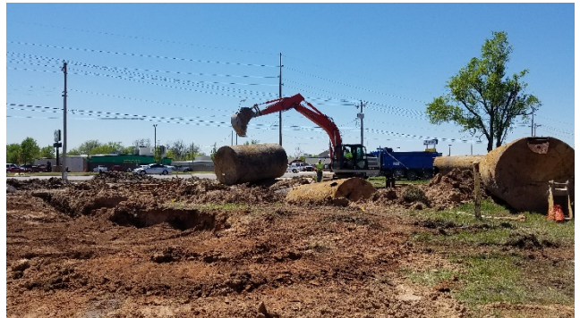
Photo #30: Tank #3 and #4 Removal
