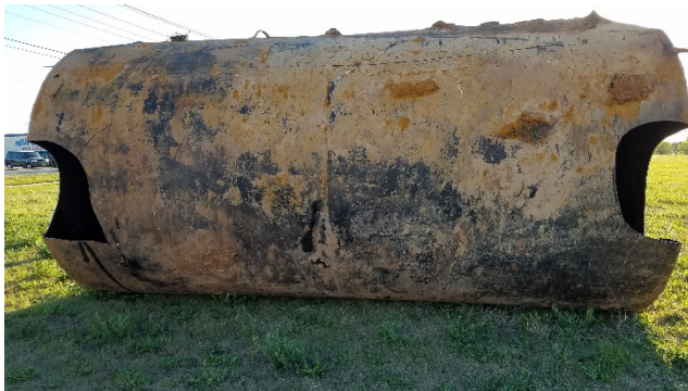
Photo #25: Larger Holes Cut in Tank #1
