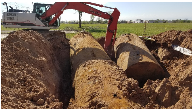
Photo #11: Tank Pit #1 : Tank #2 Removal
