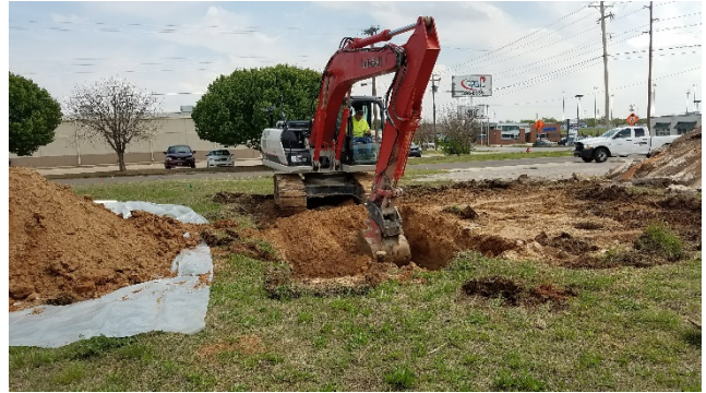
Photo #8: Tank Pit #1 : Excavation
