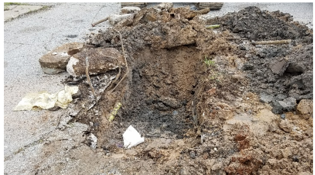
Photo #4: Dispenser Island : Removal
