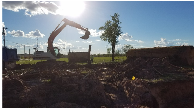
Photo #24: Hydraulic Lift Removal
