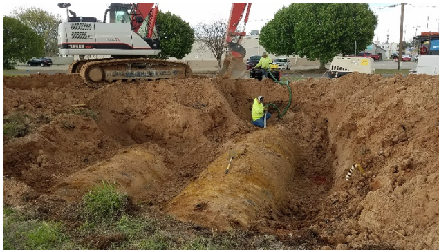
Photo #9: Tank Pit #1 : Cleaning Tanks; Tank #1 (left) and Tank #2 (Right)
