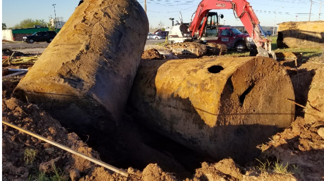
Photo #27: Tank Pit #2 : Tank #3 and #4 Removal
