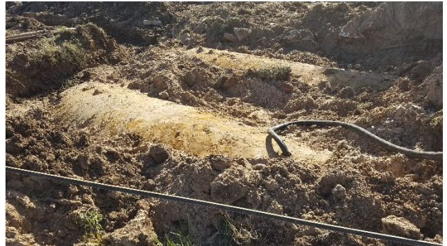
Photo #22: Removing Water from Tank #3 and #4
