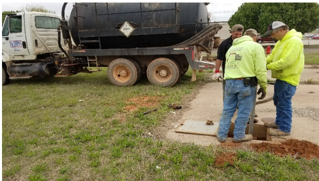
Photo #5: Water Removal from Tank #1 and #2
