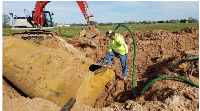
Photo #16: Tank Pit #1 : Cleaning Tank #2
