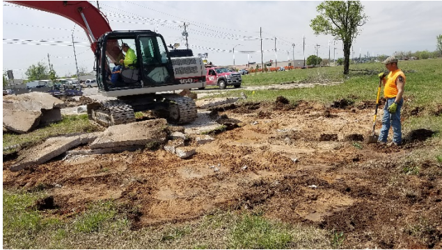
Photo #7: Tank #1 and #2 Pit Excavation
