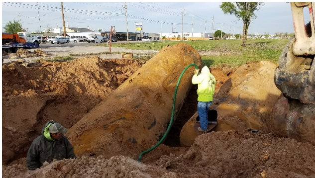
Photo #15: Tank Pit #1 : Cleaning Tank #1
