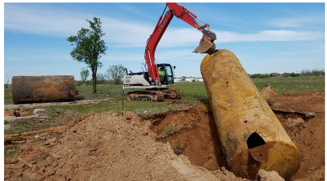
Photo #18: Removing Tank #2
