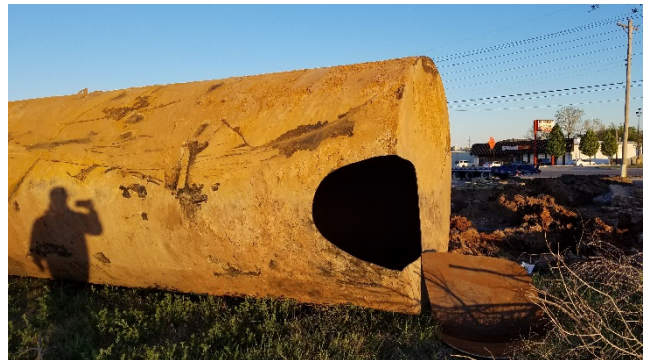
Photo #26: Larger Holes Cut in Tank #2
