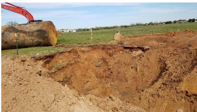
Photo #19: Tank Pit #1 : Post Tank Removal
