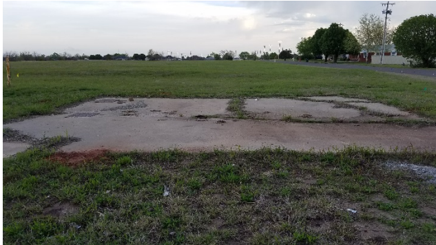
Photo #1: Tank Pit #1 : Pre-Excavation
