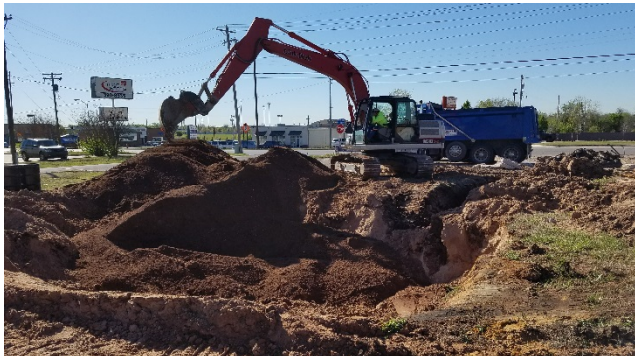
Photo #29: Tank Pit #1 : Filing in Pit with New Soil
