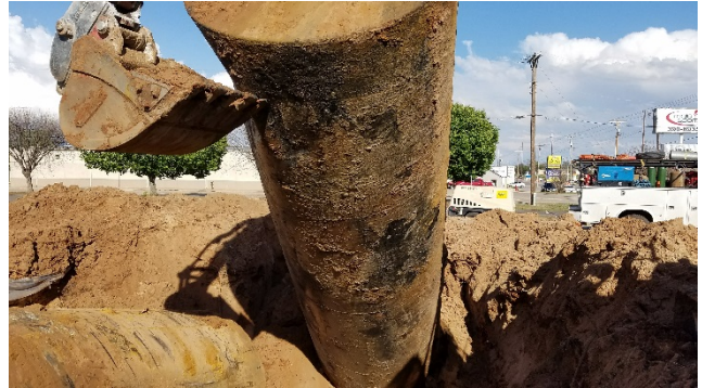
Photo #14: Tank Pit #1 : Underside of Tank #2
