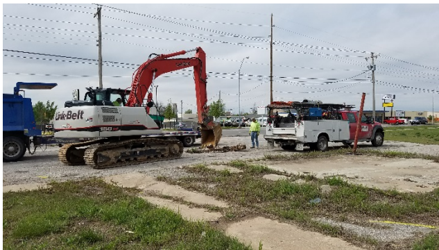
Photo #3: Dispenser Island : Removal
