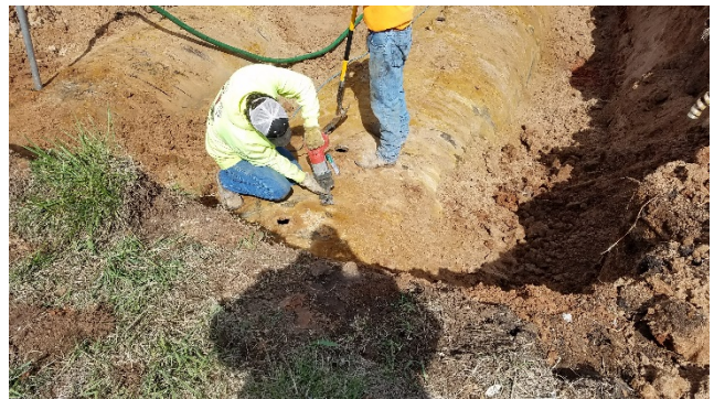
Photo #10: Cutting a Hole in Tank #2 Prior to Removal
