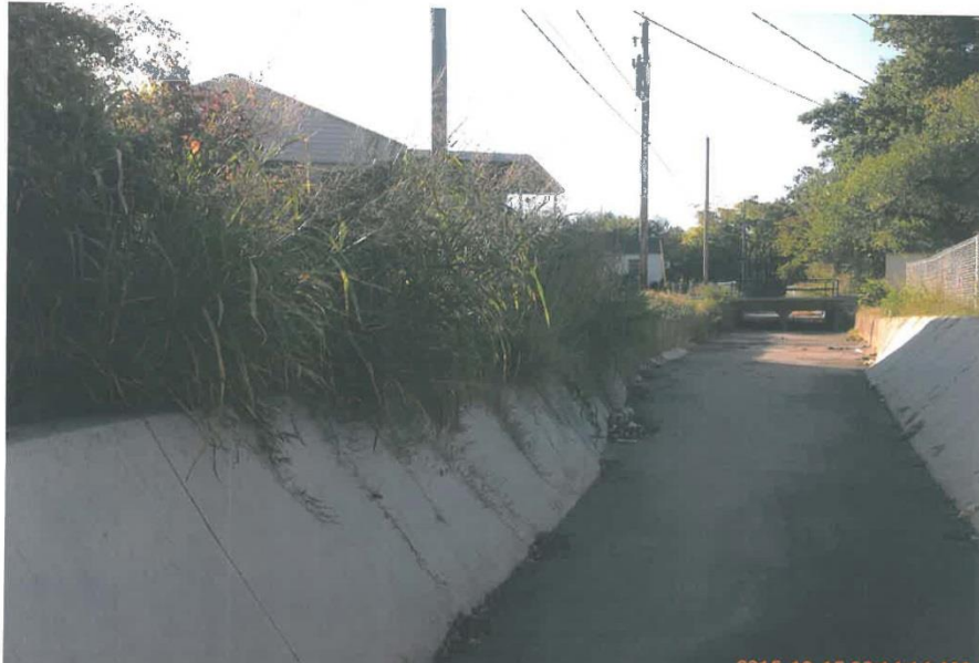
Looking toward the bridge.
