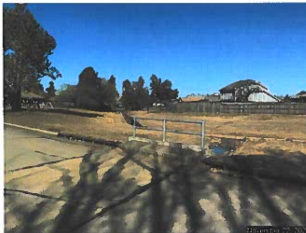
Looking north off Alicia Drive where all the drainage would cross under the road and enter Soldier Creek Tributary 6.
