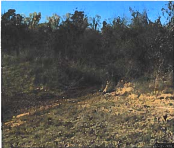
Picture of the detention outfall from Aspen 3. To the left is the beginning of the rail berm.
