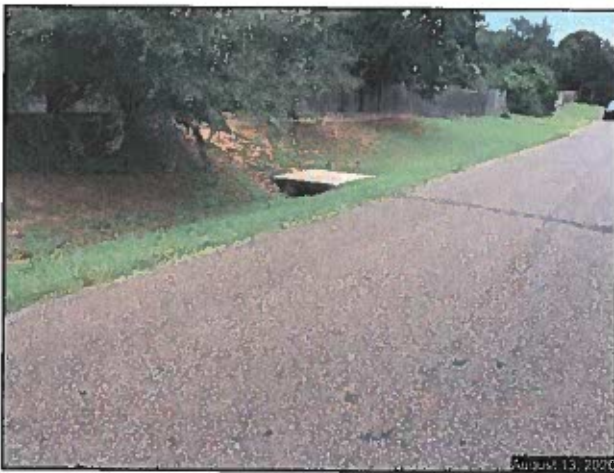
North side of SE 10 th Street, inlet catching water and Taking it via 24" pipe to east side of property in question.
