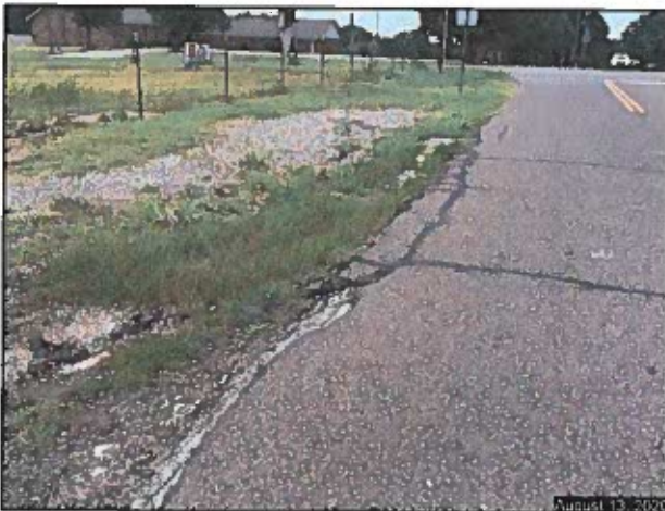
Looking west on SE 10 th Street. No curb and Gutter or Sidewalk. Note the poor condition of the roadway surface.
