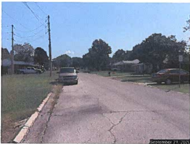
At SW corner looking east along East Jacobs Drive.
