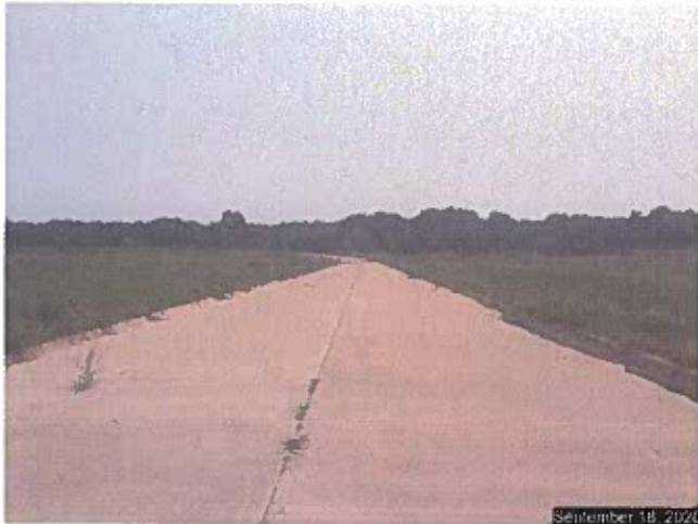
Looking south on Soldier Street.
