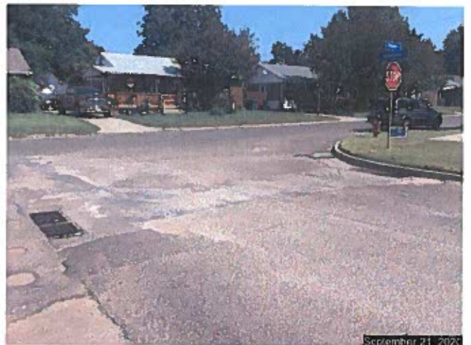
The corner of East Kittyhawk Drive and East Rickenbacker Drive. This is the upper reach of the existing drainage system. There is more infrastructure on East Kittyhawk Drive just downstream (to the west) of this intersection.
