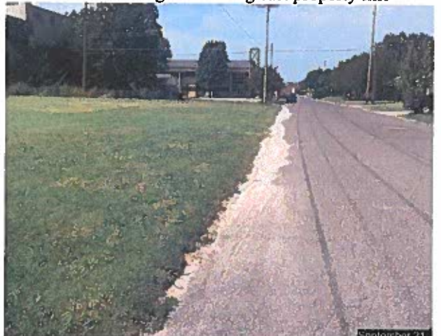
At NE corner looking west along East Kittyhawk Drive
