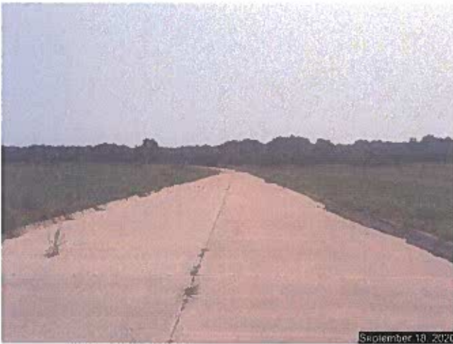
Looking south on Soldier Street.
