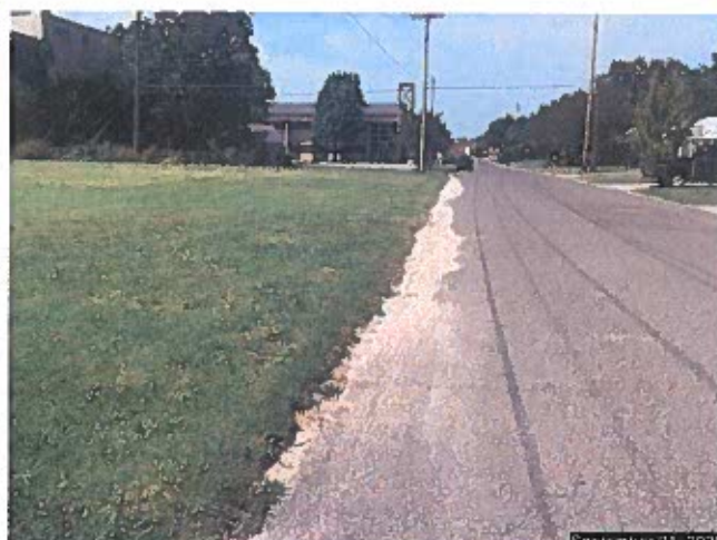
At NE corner looking west along East Kittyhawk Drive
