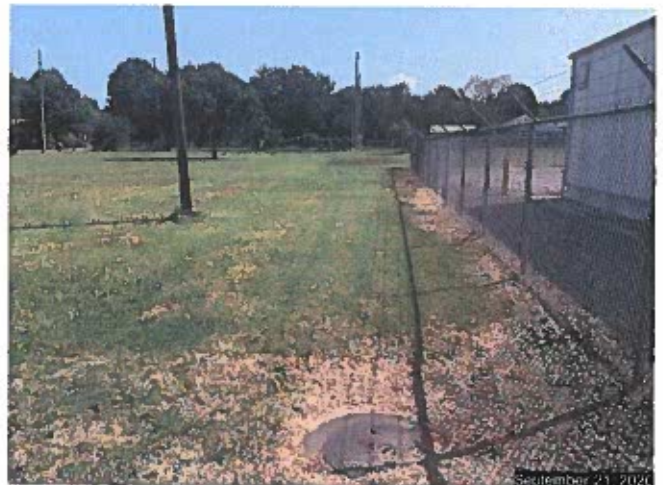
At the west property line looking east along the existing Sanitary Sewer which bisects the site
