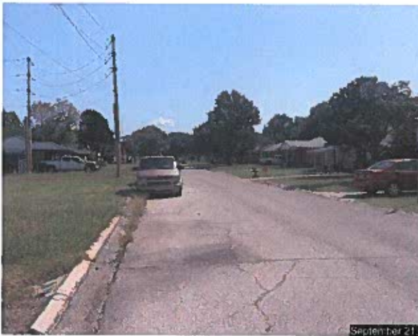
At SW corner looking east along East Jacobs Drive.
