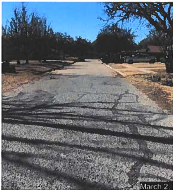
Looking west from western edge of subject plat. Shows NE 5 th Street in a city standard configuration. Concrete with curb and gutter on both sides and sidewalk
