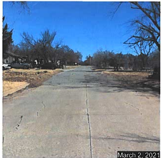
Looking east from western edge of subject plat. Subject plat is on the south side (right of picture) Shows NE 5 th Street in a city standard leading into substandard configuration along subject plat.
