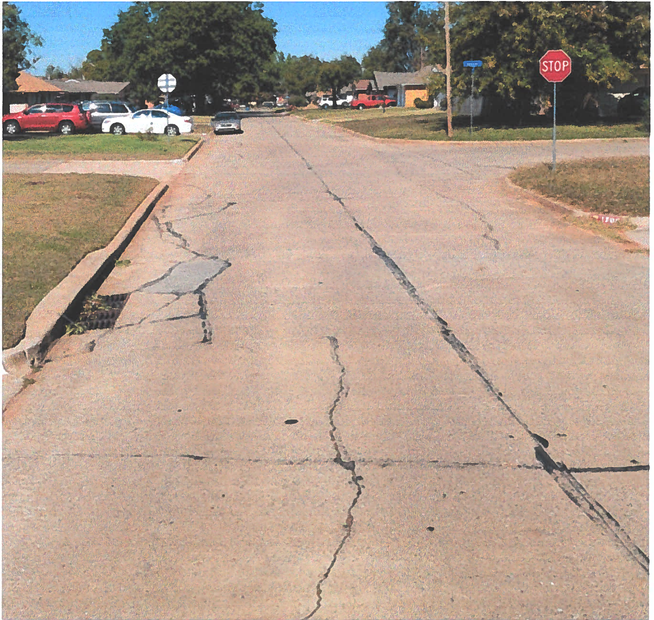
3105 N. Peebly Drive - After STOP signs were installed.
